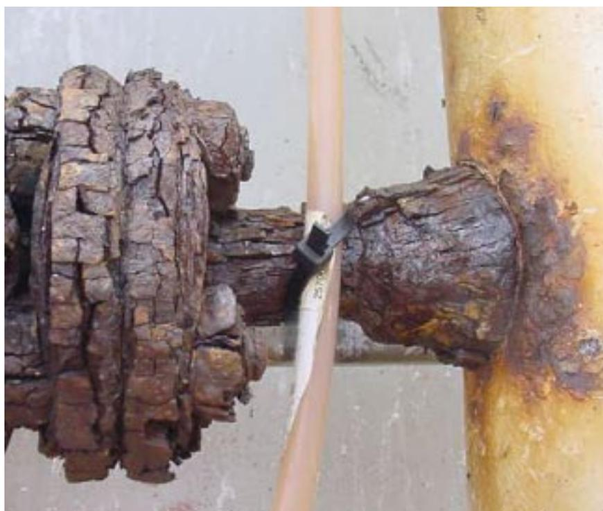
Figure 1: Lack of inspection and maintenance on a flange and bolts
